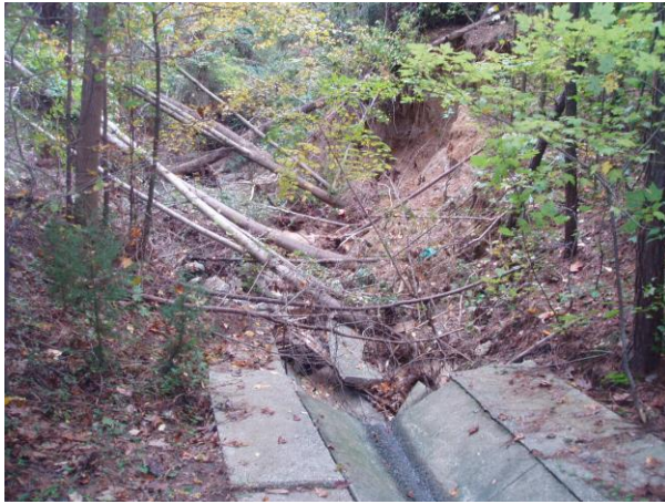
Dare Stream Restoration (Before)
