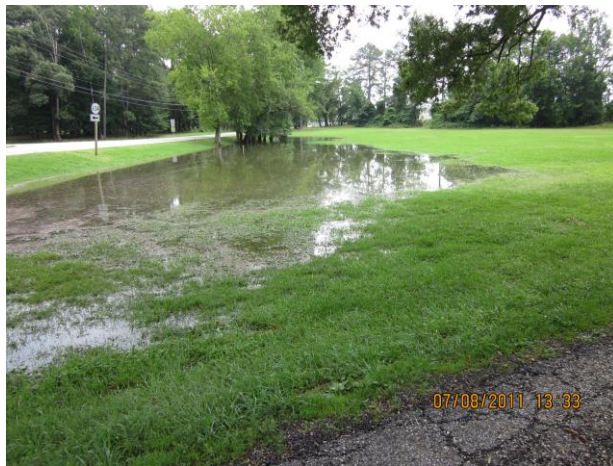
Project: Cook/Falcon Phase I (Before)
