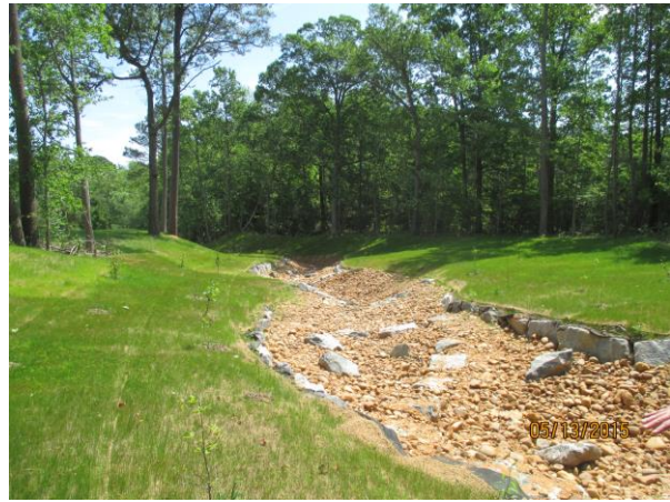
Dare Stream Restoration (After)
