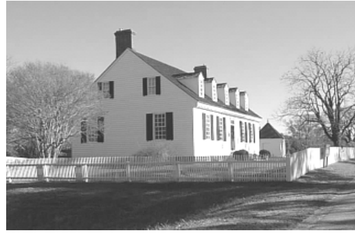
Dudley Digges House
